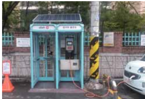
Utilizing public telephone booth as a charge station for electric vehicles
