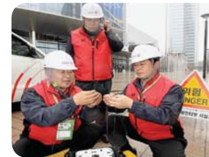
On March 23, kt staff connected optical cables near COEX in Samseong-dong, Gangnam-gu, Seoul
